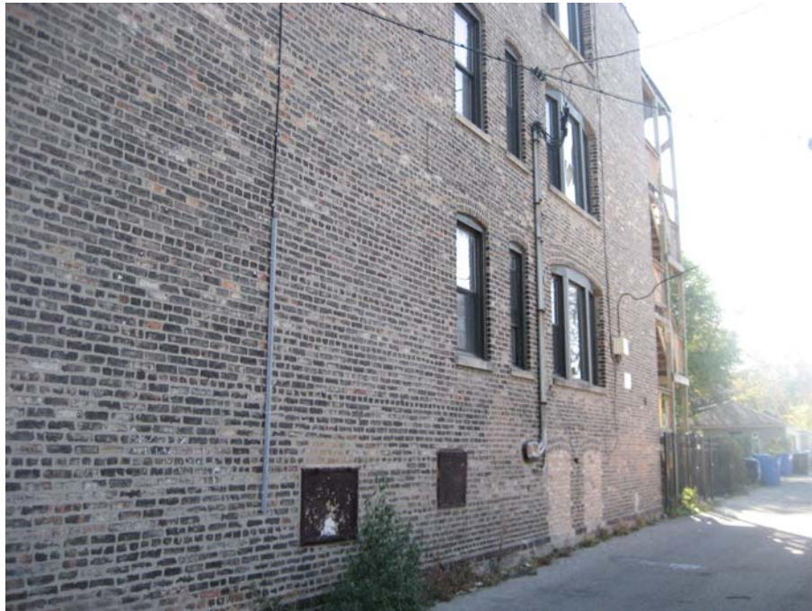
View of the western elevation looking south along a public alley
