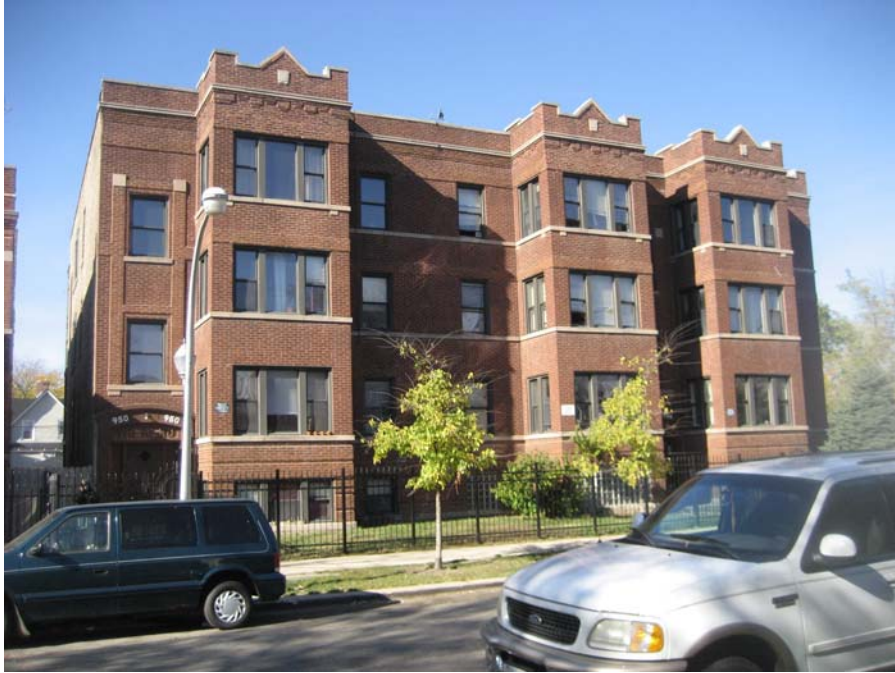
View of the subject along Laverne Avenue
