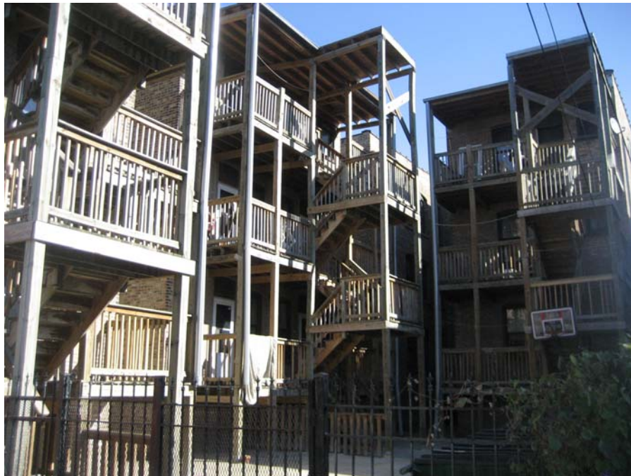
View of the rear decks
